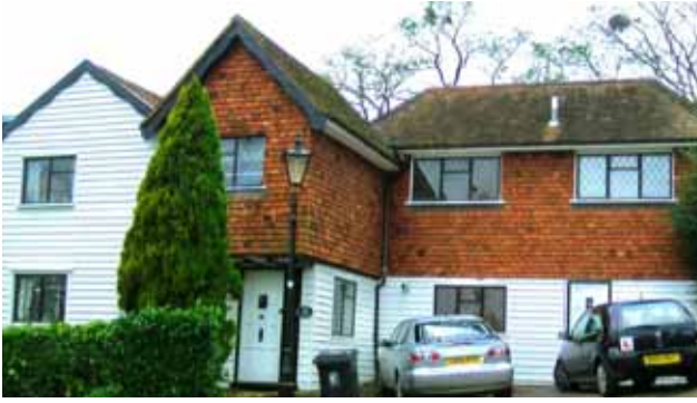
The 18 th -century Alma cottage at the corner of Steeds Way and York Hill was enlarged and mostly tile hung
