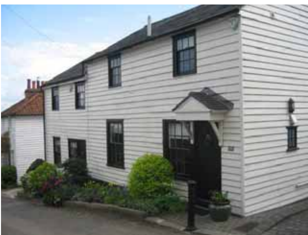
This pair of early 19th century cottages at 19 and 21 Forest Way were extended late 19th century. They are timber framed, weatherboarded and roofed with hand made clay tiles . There is a central chimney stack between the two cottages.
