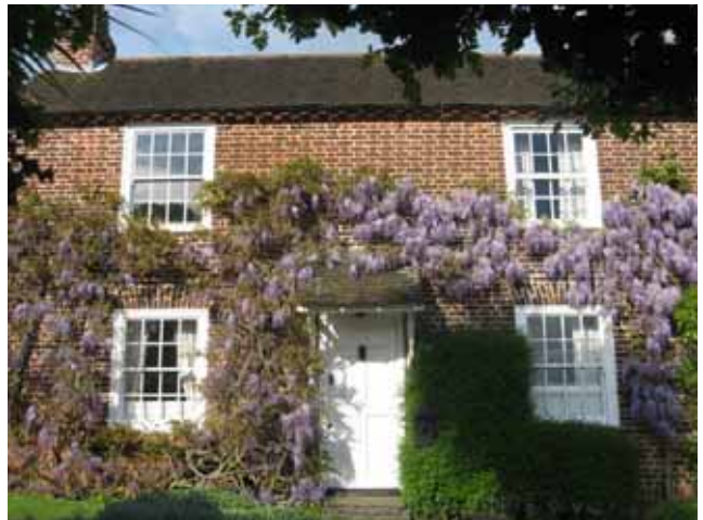
107 York Hill is an 18th Century red brick house, Flemish Bond roofed with handmade red clay tiles.
