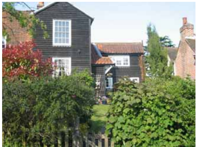
109 York Hill is two cottages combined to form one and built in the late 18th century.
