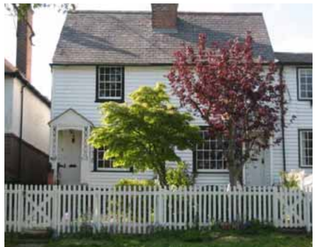
Below: The early 19th Century cottages on School Green—34 and 36 York Hill—are timber-framed, weatherboarded and roofed with slate pictured 100 years ago (below left) and now.
