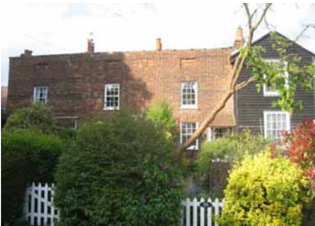
The terrace of three cottages at 111, 113 and 115 York Hill distinguished by a parapet concealing the roof.
