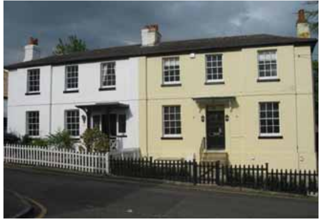
19 and 21 York Hill, next to The Wheatsheaf have recently undergone sensitive restoration, keeping the traditional wicket fences.
