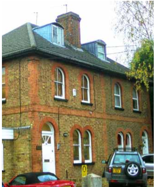
such as fences and hedges be brought into line with the neighbouring Staples Road Conservation Area to cover materials used on road frontages. Slate roof with dormer windows; cheaper yellow brick edged with harder red brick on edges and around windows. 16-18 York Hill
