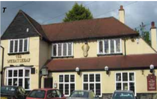
The Wheatsheaf has changed dramatically over the centuries but still provides an imposing facade at the entrance to the York Hill Conservation Area
