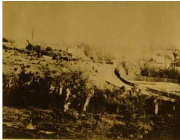
Staples Road pictured in 1877 showing the lopped trees: a very different picture from today.
