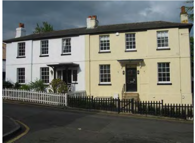
19 and 21 York Hill, next to The Wheatsheaf have recently undergone sensitive restoration, keeping
