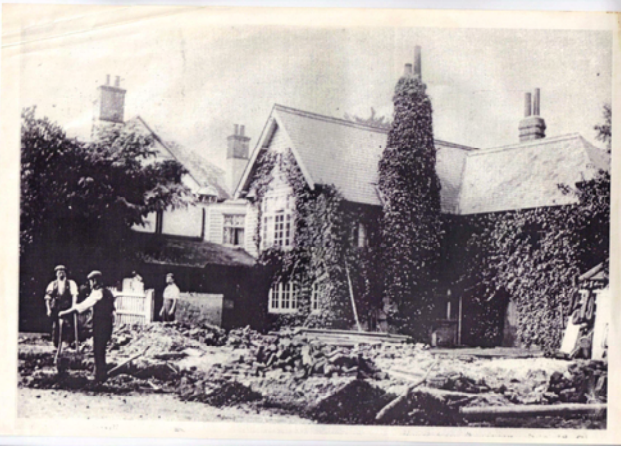
Ash Green House reconstruction in the early 1900s
